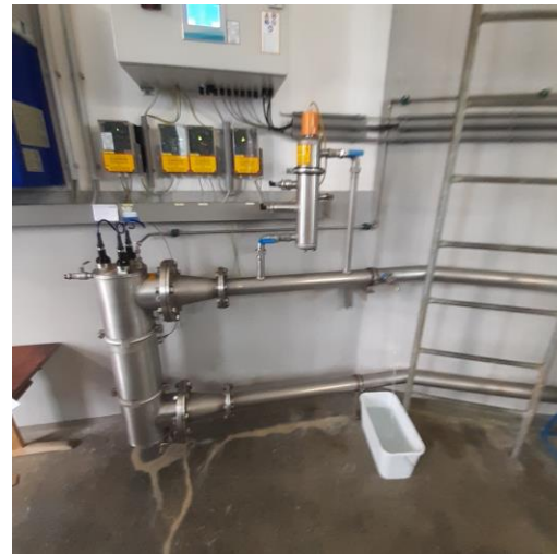
Abb 5: UV-Anlage (Br. I+II+III)
