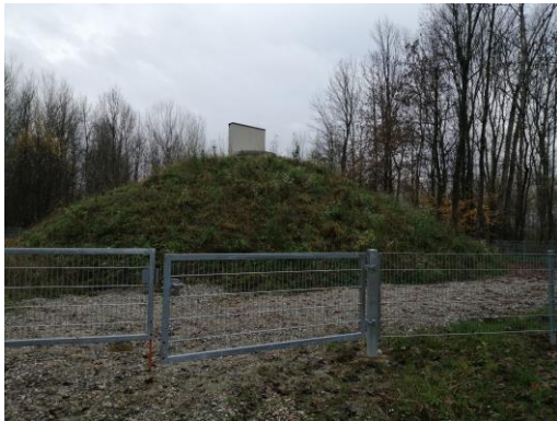
Abb. 1: Neuer Bohrbrunnen "Au"
